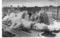
1. Pruitt-Igoe demolition. Courtesy of U.S. Army Postcard Co.
