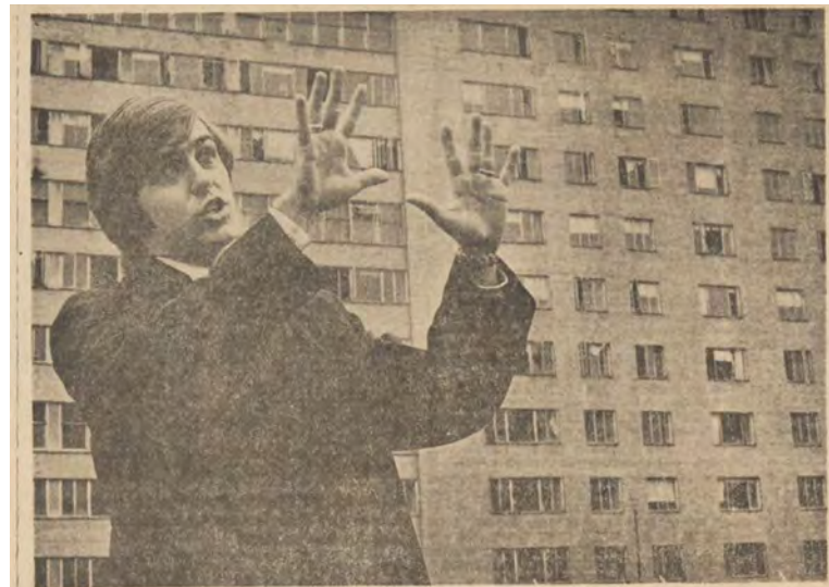
AN OUTLINE OF DEMOLITION being shaped by the hands of J. Merk Loizeaux of Baltimore as he explained an experiment in cutting stories off the tops of buildings in the Pruitt-Igoe housing complex. (Post-Dispatch Photo)
